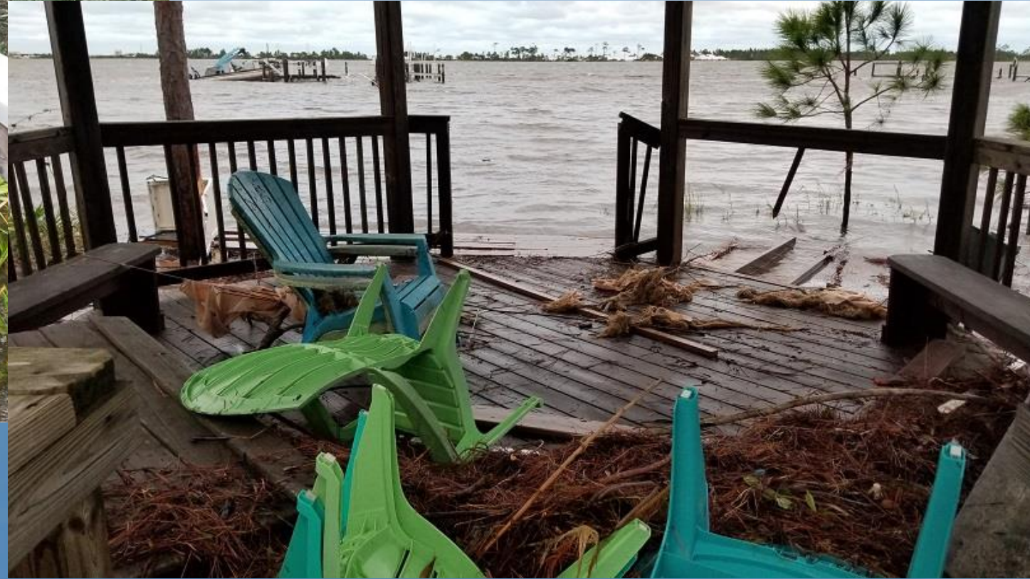
Gazebo and Dock Repairs
